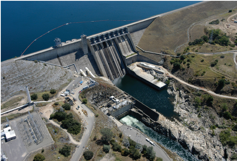
Folsom Dam is a concrete gravity dam along the American River in California.
