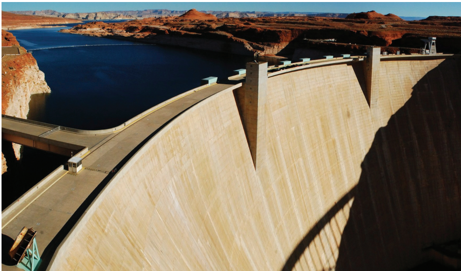
Glen Canyon Dam is a concrete arch dam on the Colorado River in Arizona.
